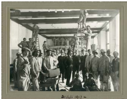
Bau Le Restaurant 1913 Badrutt's Palace Hotel Archiv
